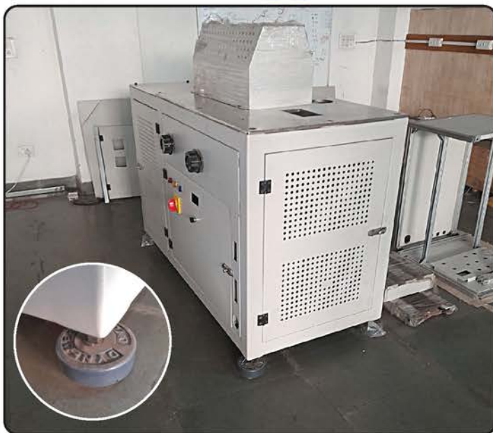
Panel on Dynemech Round Mounts, Series DLC
