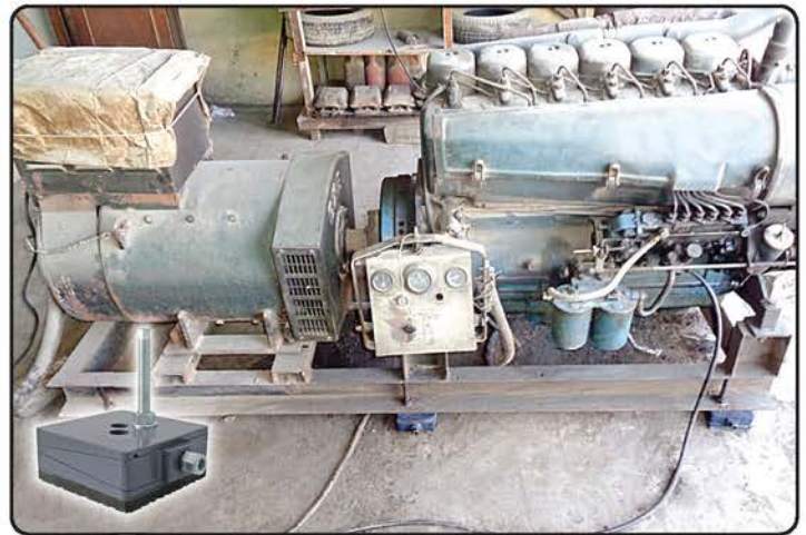
DG Set on Dynemech Wedge Mounts
