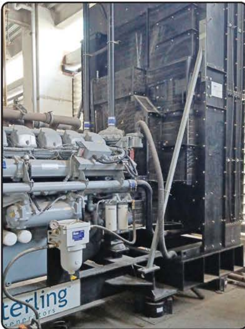
Genset on Dynemech Spring Isolator with Viscous Damping
