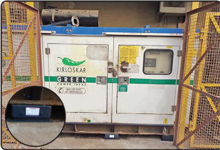
Genset on Dynemech Spring Isolator with Viscous Damping
