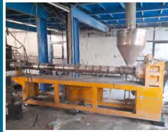
Extruder Machine installed on Spring Isolator MDI
