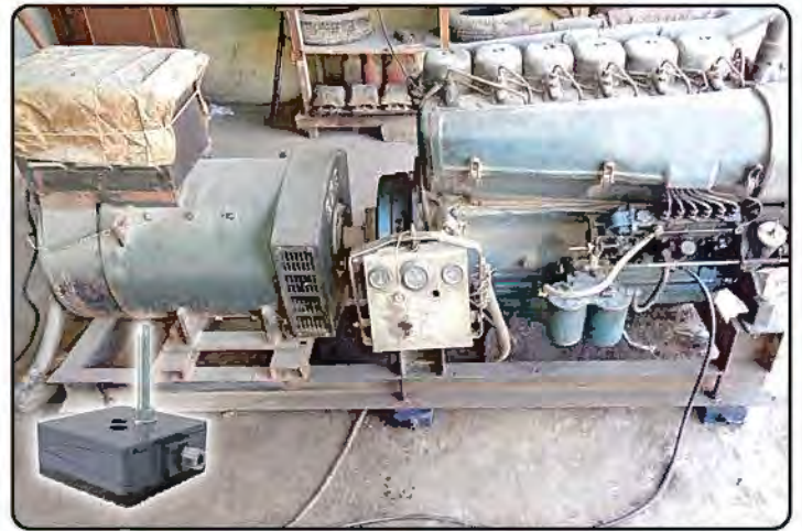
DG Set on Dynemech Wedge Mounts
