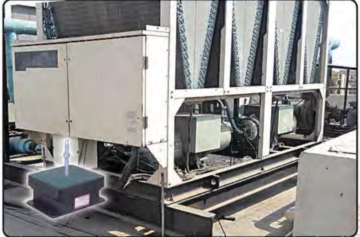
Chillers on Dynemech Spring Isolators with Viscous Damping
