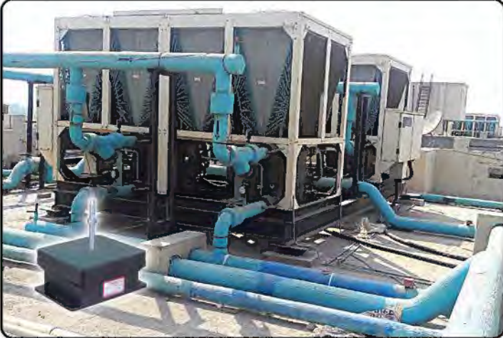
Chillers on Dynemech Spring Isolators with Viscous Damping
